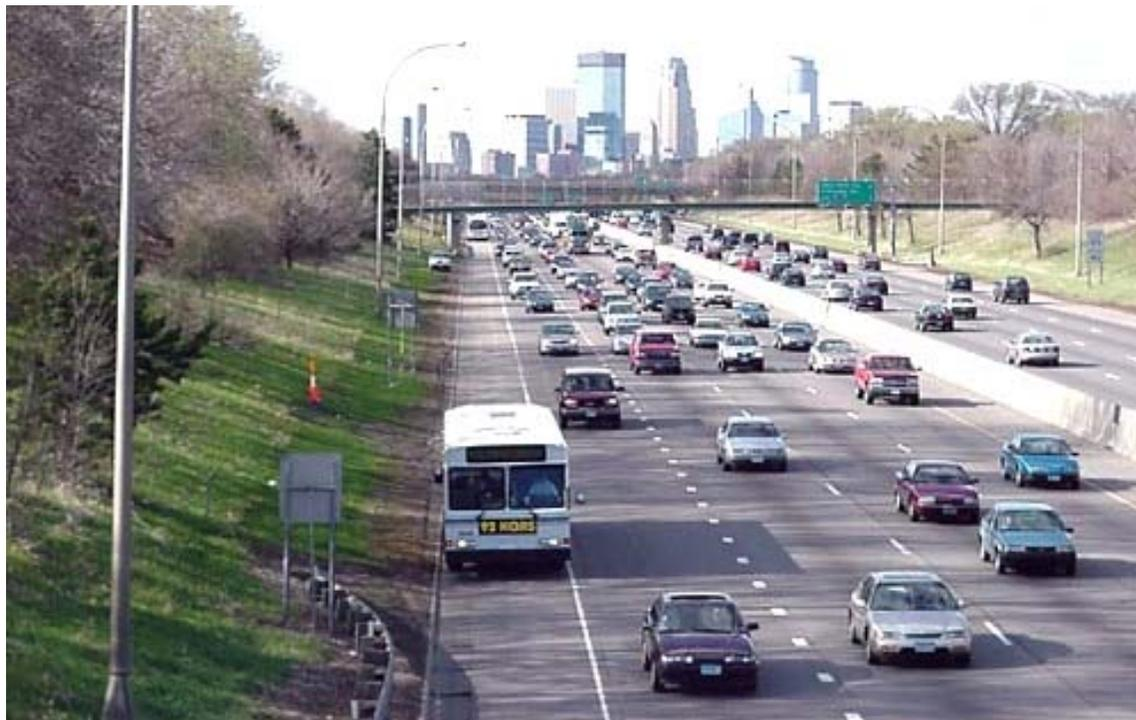
not permitted to operate more than 15 mph faster than the general traffic lanes. To better facilitate bus operations on highway shoulders, Metro Transit and the Minnesota Department of Transportation are widening highway shoulders throughout the Twin Cities area (to 12 feet where possible).
